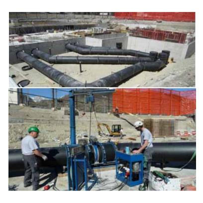
Material: PE SDR33 welded
